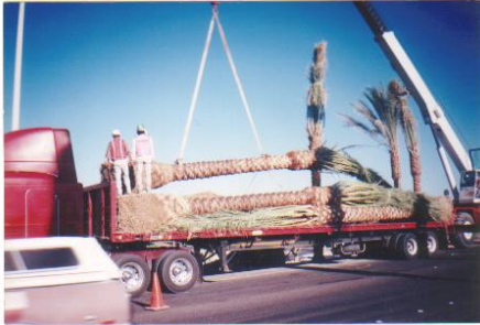
Figure 7-Palm rigged to be picked horizontally with nylon slings
