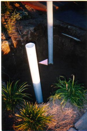
Figure 11-Drainage manifold installed into planting pit
