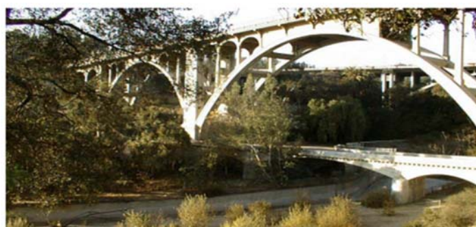
Parker-Mayberry Bridge below the Colorado St. Bridge
